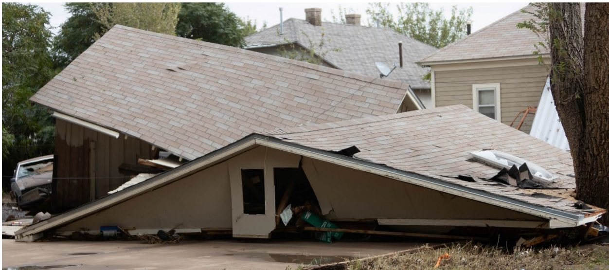
Figure 10: Image of Post-Flood Home Damage (Chaves County). Photo Credit: Juliana Halverson
