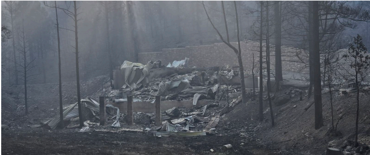
Figure 9: Image of Post-Fire Home Damage (Lincoln County).
