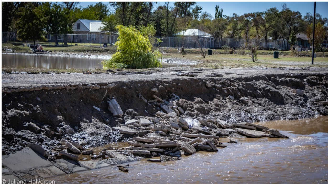
Figure 11: Image of Waterway Damage (Chaves County). Photo Credit: Juliana Halvorson
